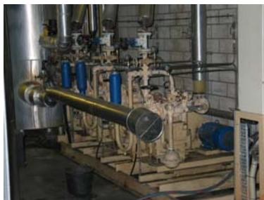
Since her start in 1930 Clayton applies the counter flow principle for the heat exchanger which guarantees maximal thermal efficiency. The boiler water is enclosed in a long steel pipe which is spirally wound into a helical coil.
