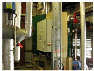
Generator, Feedwater Treatment Skid and Feedwater Booster Pump. The Feedwater Treatment Skid includes the Horizontal Hotwell, Water Transfer Pumps and Blowdown Tank piped and wired to form a packaged water system.
